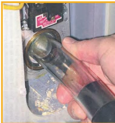
(l-r) A universal hose adaptor. Three-feet of one-inch inside diameter vinyl tubing. Vacuuming through element opening.
