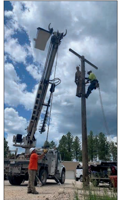
BHEC crews demonstrating pole top rescue techniques.
